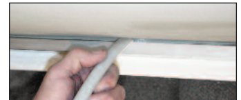
STEP 5: Pour in Expansion Cement to 3/8" (9.5 mm) below the top. Allow adequate time for it to set.
